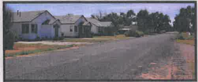
Street in Walsh, Colorado, that was repaired doing Full-Depth Reclamation with their Asphalt Zipper® and then chip-sealed.
