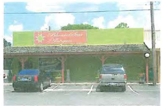
Stucco is not historically a common material in Blanco.
