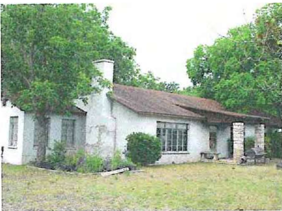
Chimneys are an important architectural feature that should be maintained and repaired when necessary.
