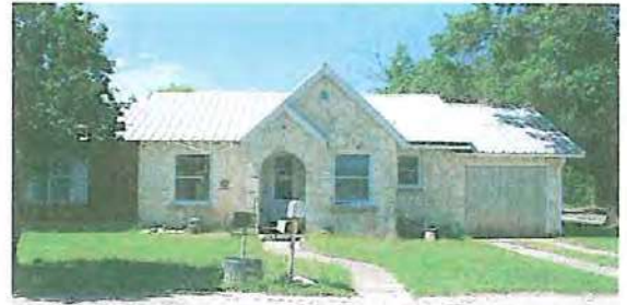
Residence with an addition to the left side.
