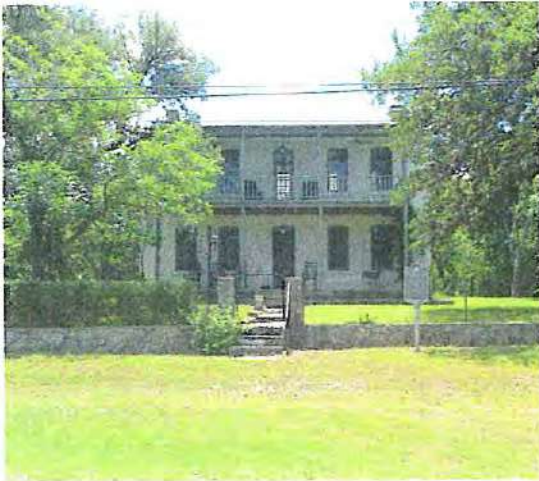
Historic residences have different proportional relationships, such as high ceilings with tall windows.
