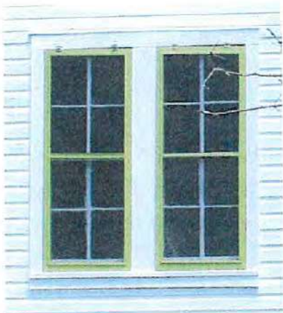
Maintenance to wood windows can substantially improve the energy efficiency.
