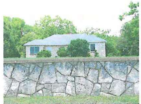
Stone is also used for retaining walls and planters throughout Blanco. This wall is random field stone.
