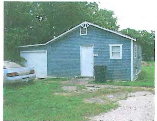
Over time, dark colors begin to look faded and chalky. If selected, they must be more regularly maintained.
