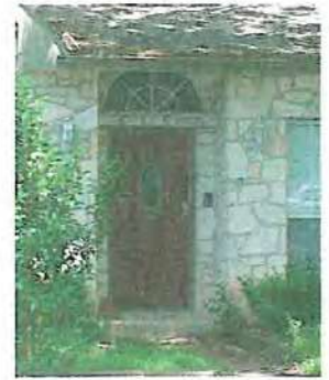
Above the entry door is an example of a fanlight.
