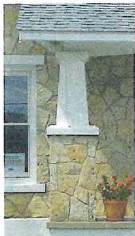
A tapered box column with a masonry base.
