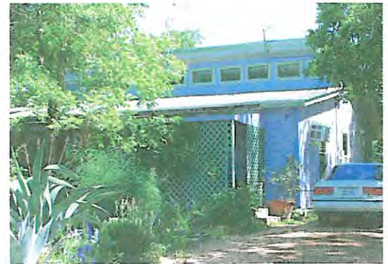
A row of clerestory windows between the two roof-lines.
