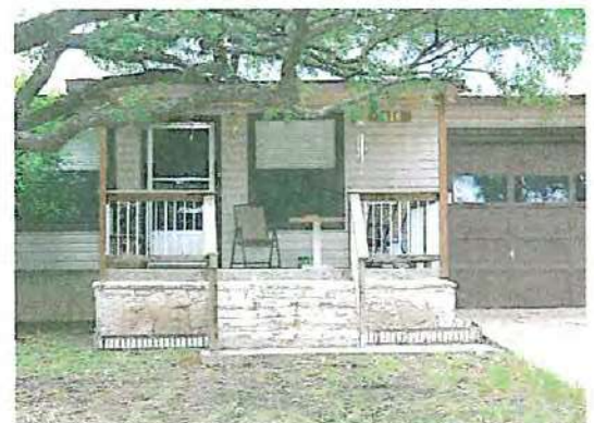
A porch railing with spindles .
