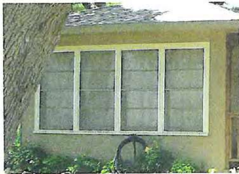
A series of windows with mullions between each window.
