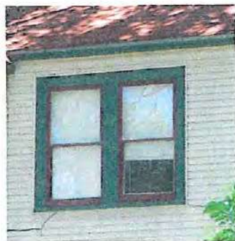
An example of a window in a one-over-one configuration.
