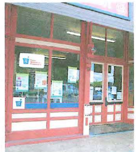
A cast iron commercial facade.
