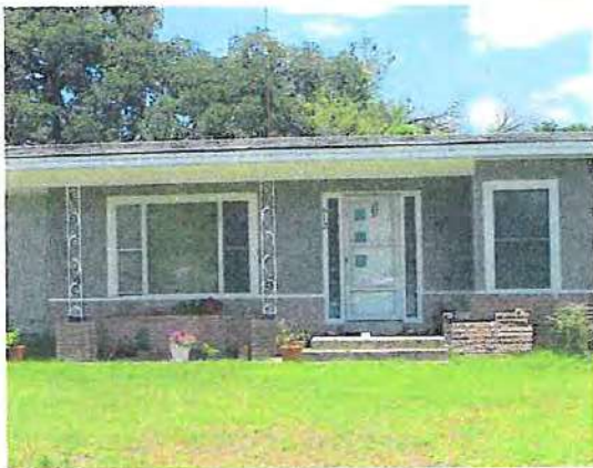
An entrance door with side lights.
