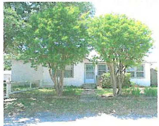
Avoid installing siding of a different scale or profile than the original siding.
