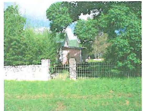
Stone walls should be retained.
