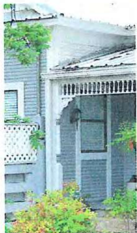
An engaged column on a porch.
