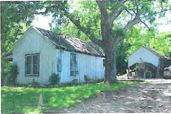
A residence with board-and-batten siding .
