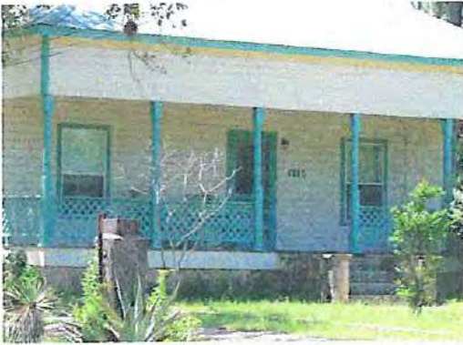
A balustrade with wooden lattice .
