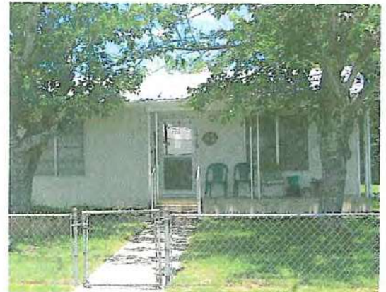
If adding a storm door, choose a "full vision panel" to allow the original door to be seen.
