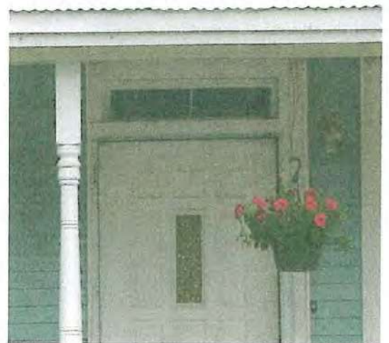
Retain and repair, if necessary, original transoms.
