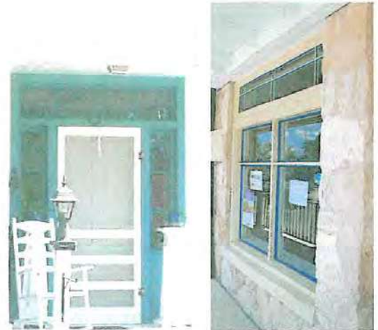
Left: An entry door with side lights . Right: A solid sill located at the bottom of the window.
