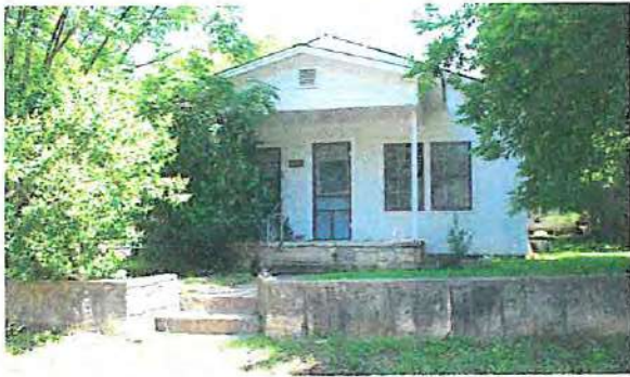
The retaining wall with stairs helps define the front entrance.
