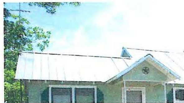
A residence with v-crimp roofing .
