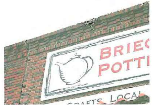
Brick is used for decorative features, which should be preserved.
