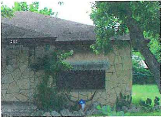
When adding shading devices, they should be appropriately proportioned and be consistent with the house's character. The above shading device is inappropriate for this house.
