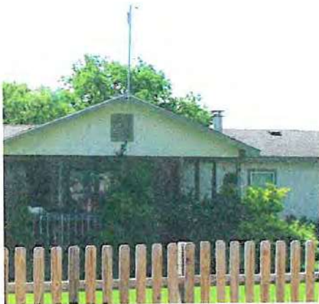
Modern amenities, such as the antenna, should not be located on the prominent or street facing facades.
