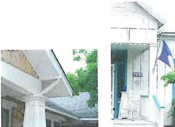
Left: A wooden bracket at the eave. Right: A porch with a box column .
