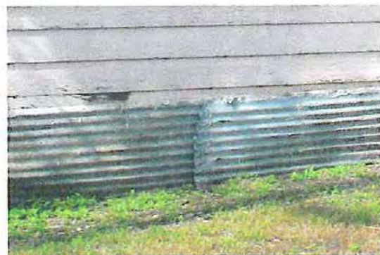
Metal materials should not be used to replace non-metal materials on buildings.
