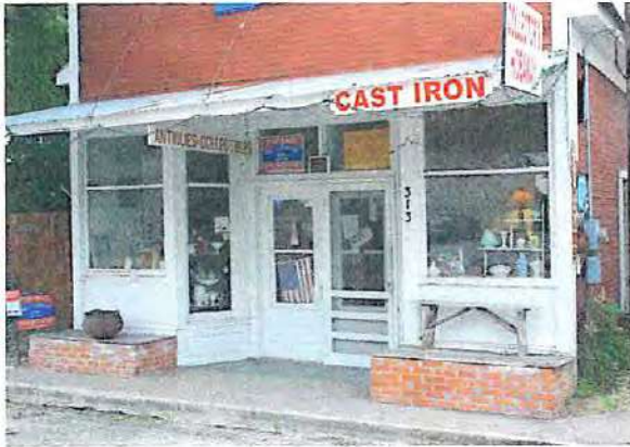
A commercial building with a wood facade and parapet.
