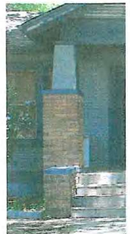
An example of a brick column base.
