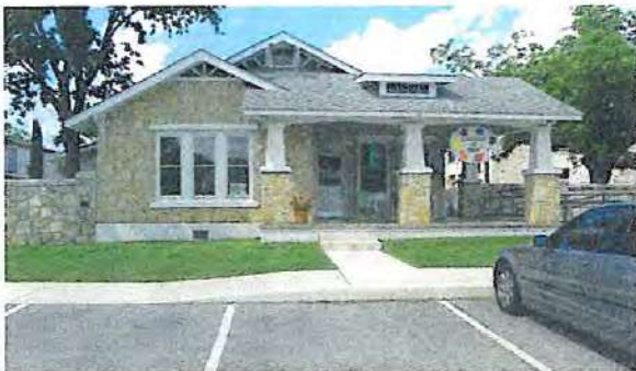
Stone is a predominant building material within Blanco.
