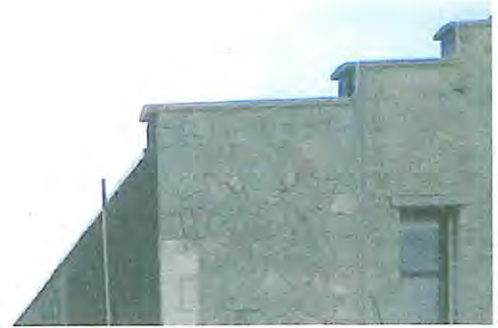
A parapet along the front facade.
