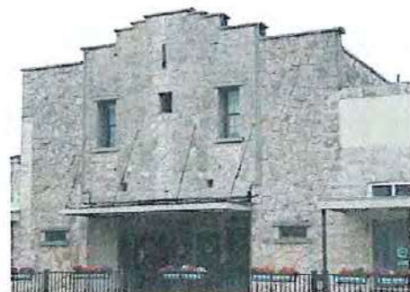
A canopy with rods at the building's entrance.
