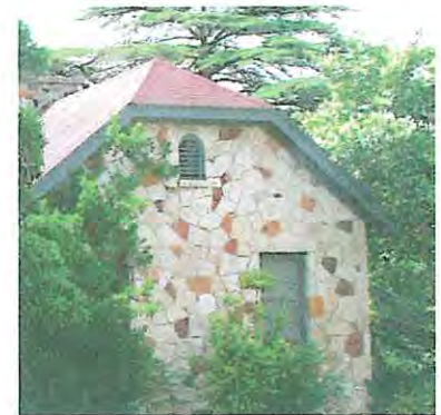
An example of a clipped gable on a roof.
