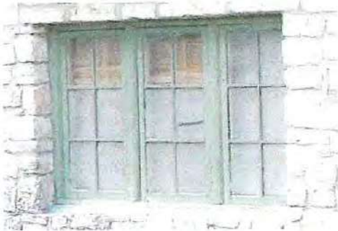
A divided light sash on a residence.
