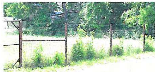
A fence consisting of welding wire fencing .
