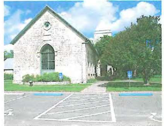
An example of a cut coursed stone building.
