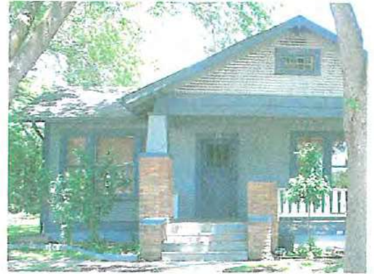
When replacing doors, the design should be consistent with the style and era of the residence.
