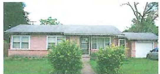
Asbestos shingles do not cause irreparable damage to underneath materials.
