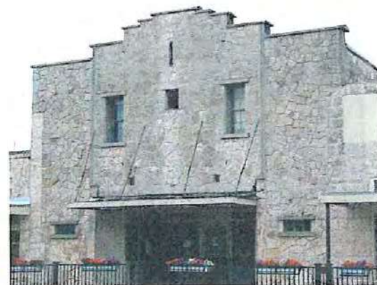
Example of canopies hung using rods.
