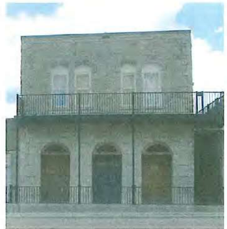
Replacing missing cornice and details is encouraged when enough evidence exists.
