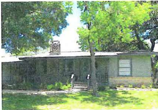
When adding an access ramp, it should be thoughtfully placed and designed within its context.
