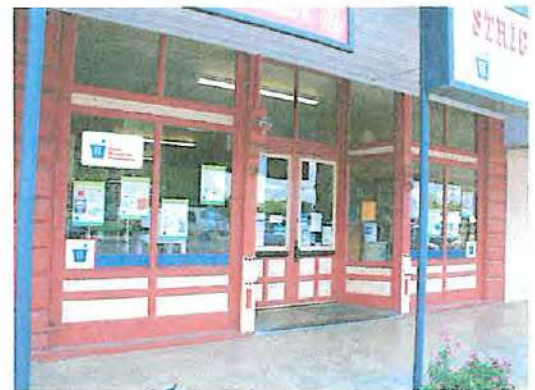
Similar kick plate design on doors and the front of store.
