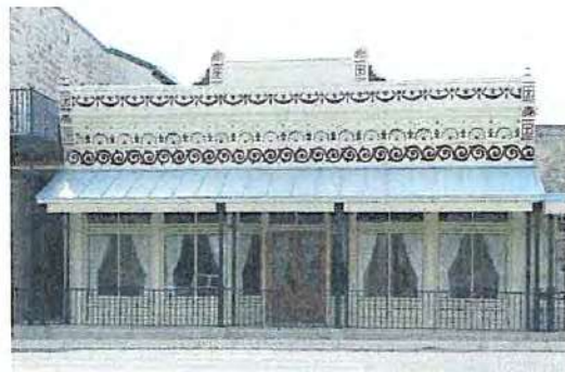
Detailed cornice at roof line retains its historic character.
