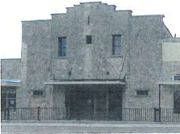
Example of tall, narrow windows that appear to be “punched” out, these should be maintained.
