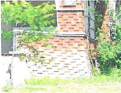
Flared shingle skirting example on a craftsman residence.
