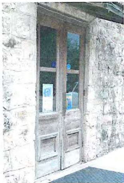
Historic doors should be retained and repaired when necessary.
